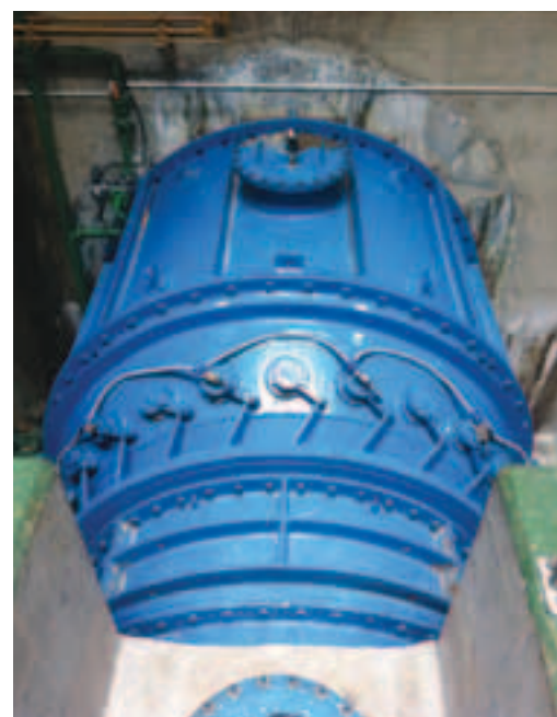
The Kaplan-type turbine used for the Sol Plaatje and Merino installations.
