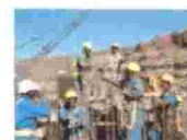
Workers at the Sol Plaatje project
